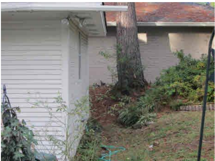
VIEW ALONG THE BACK OF THE MASTER BATHROOM WING FACING 13634 PINEROCK
