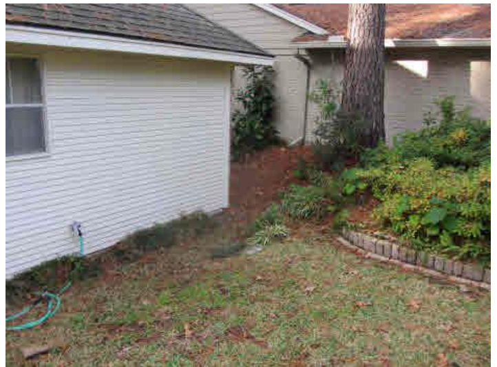
REAR VIEW OF THE MASTER BATHROOM: NOTE THE HIGHER GROUND RIGHT BEHIND THE HOUSE IS THE FAULT ZONE
