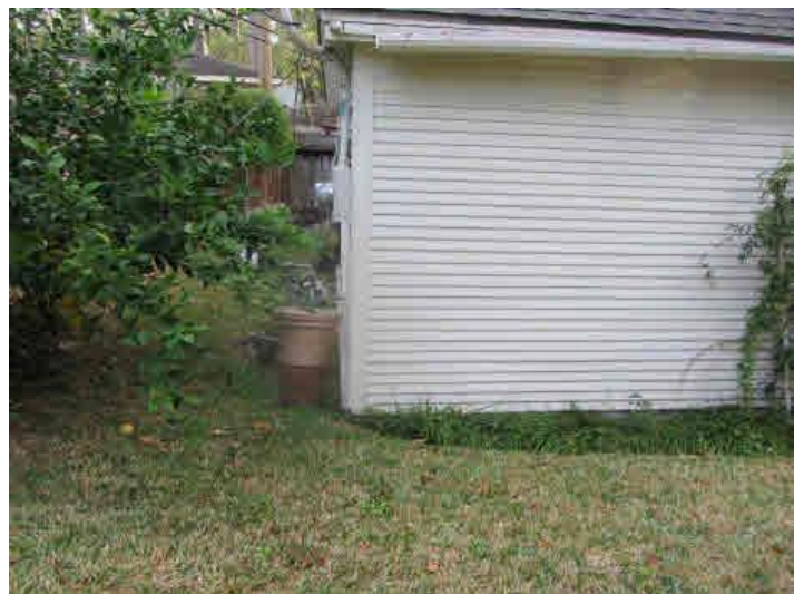
VIEW OF THE AREA BEHIND THE TWO CAR DETACHED GARAGE
